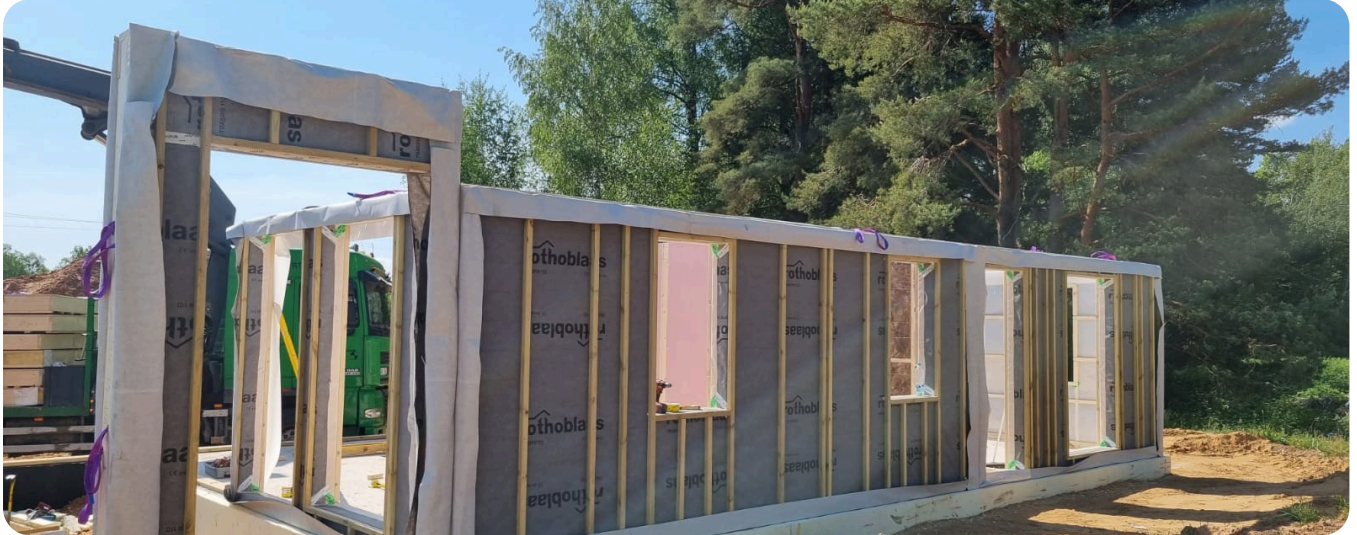
Panels being erected on site · factory reference project
