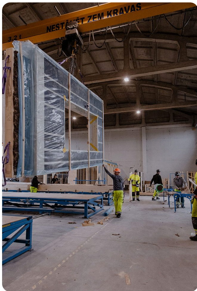
Wall panel in the factory, Birzgale
