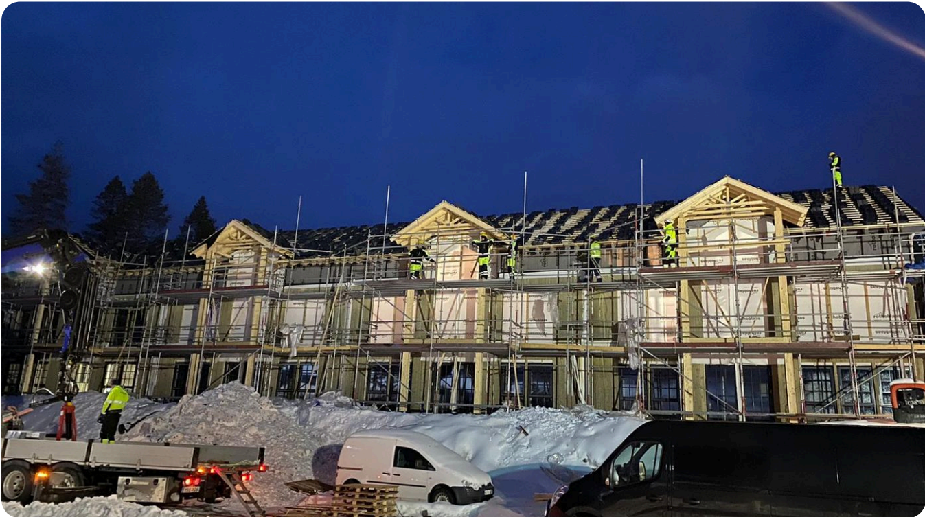
Idre, Sweden · factory reference project, during assembly
