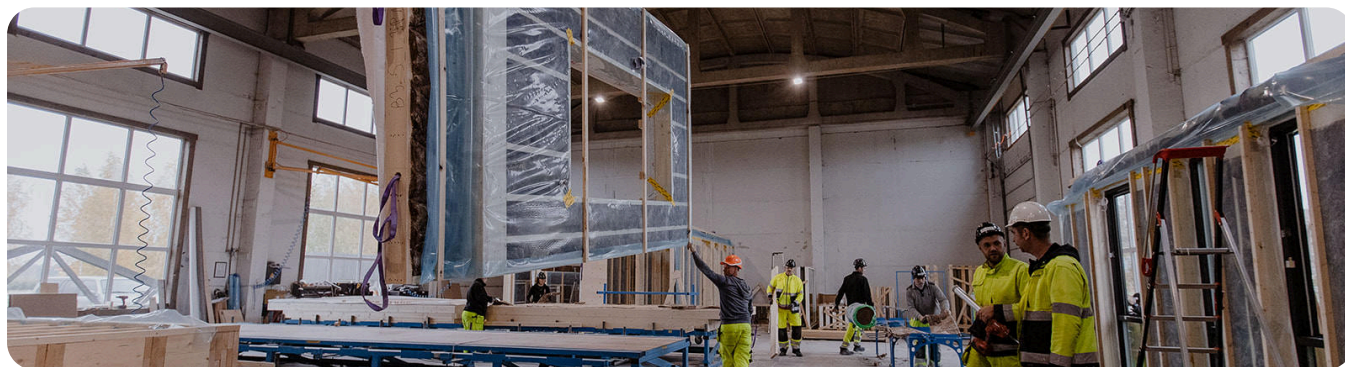
Wrapped wall panel on the factory's gantry crane
