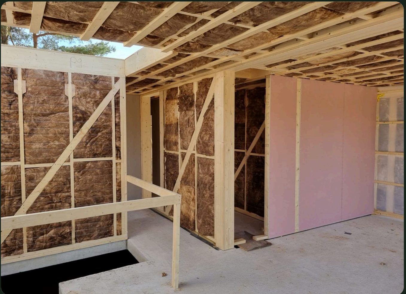
Panels assembled on site, before interior finishes · factory reference project, Latvia
